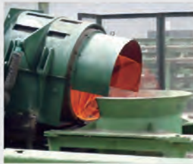
Production line for heavy coil
